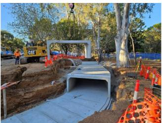
The project involves the replacement of the existing twin cell culvert beneath Unley Road that facilitates the flow of Park Lands Creek from Park 19 into Park 20. The existing culvert is in poor condition with walls being held up by props at the western end.
